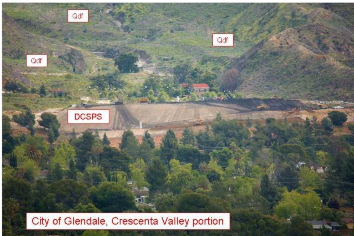
Figure 4. Outlet channel for Dunsmore debris basin (debris dam and basin are located behind vegetation). Looking north from point where channel passes under Markridge Road: a potential debris-flow spreading point if basin fills and excess flow continues into channel.
